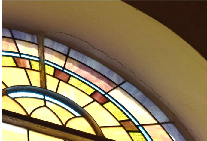
Figures 5.28 and 5.29: Weathered floor near the entrance threshold. Cracked plaster near a window header on the east wall.
