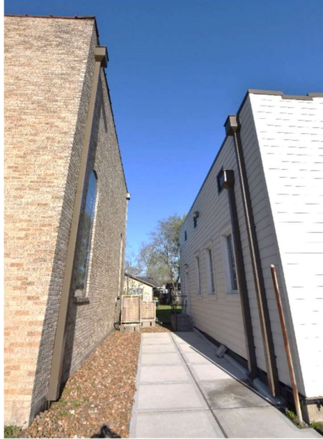
Figure 5.30: Area between the north end of the sanctuary and the detached hall. This area is also visible at the right of Figure 5.11.
