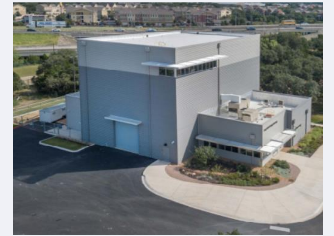
Fig. 1 - Large Scale Testing Laboratory
